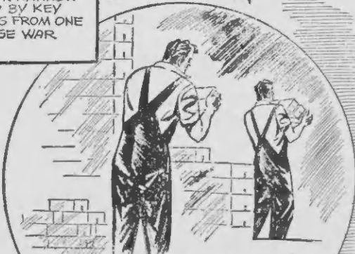
THE DEVELOPMENT OF SLOTTED GLASS BLOCKS REQUIRING NEITHER NAILS NOR FASTENERS MAKES POSSIBLE INTERIOR WALLS THAT CAN BE MOVED OR CHANGED IN SIZE
